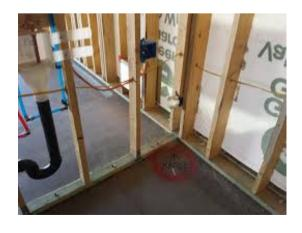
Before the drywall goes up, it is a good idea to take pictures of where extra blocks, pipes, electrical wiring (and so on) could interfere in the future when you want to hang artwork, TV's and such.
